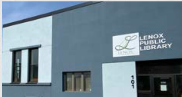
Pictured left, newly renovated exterior
